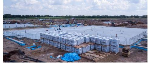
STORAGE: Pallets will arrive at job on pallets shrink wrapped and with a pallet cover. Place pallets in original shipping packaging on high point of area so no rain will puddle around the pallet and so air will flow underneath. No need for storage containers if stored onsite in this manner.
